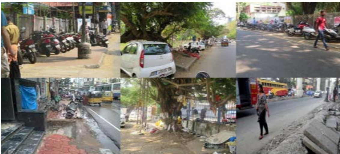
Figure 39 - Obstructions in the form of debris dumped, vehicles parked, light pole and trees, damaged slabs on the footpath
