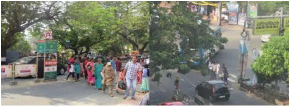
Figure 38 - Pedestrian struggling to cross the road, faded zebra crossing at High Court Junction
