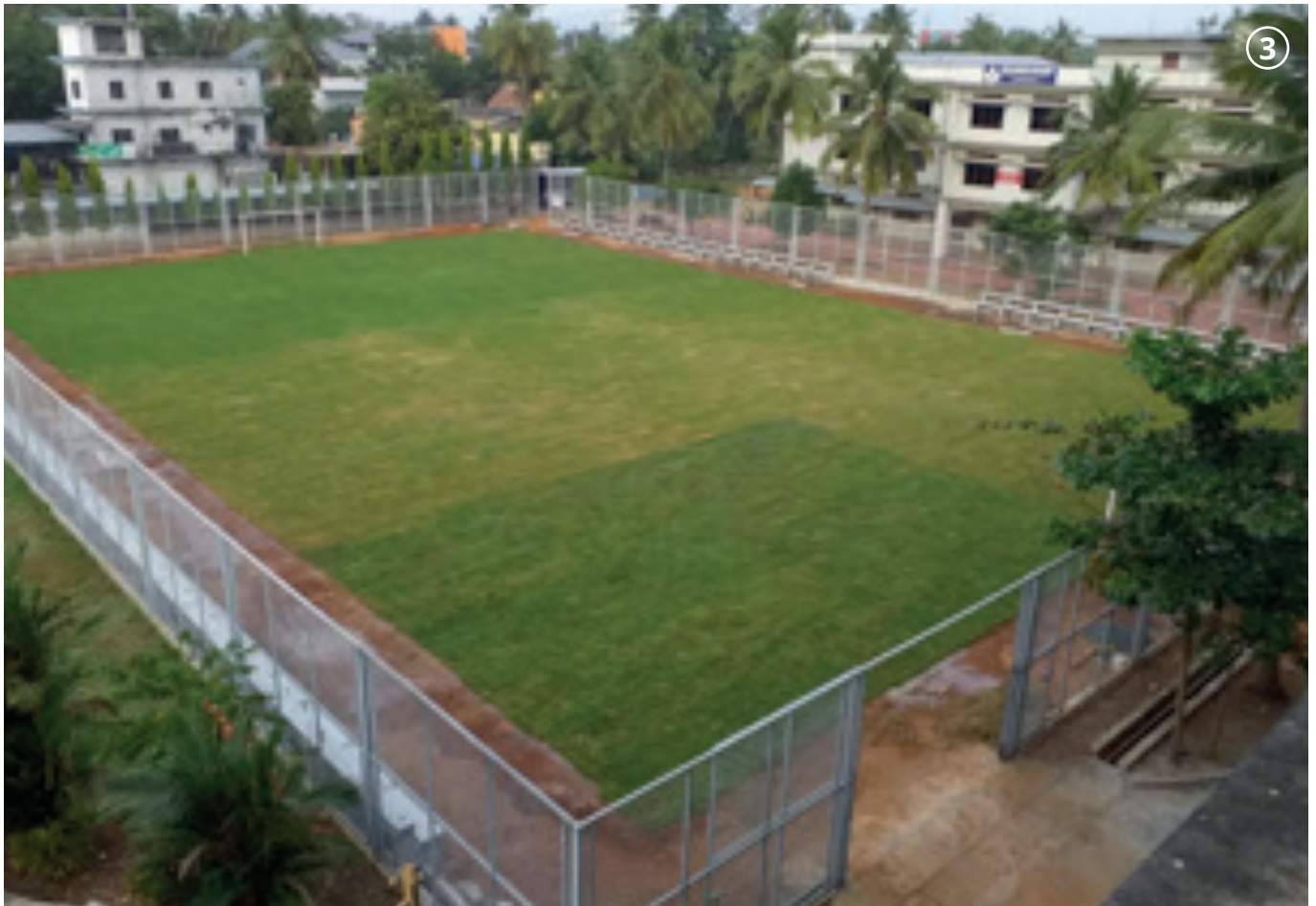
Picture 1&2 - Basketball court and badminton court constructed at CA High School, Ayakkad, Kerala Picture 3 - Football court constructed as part of CYRC project
