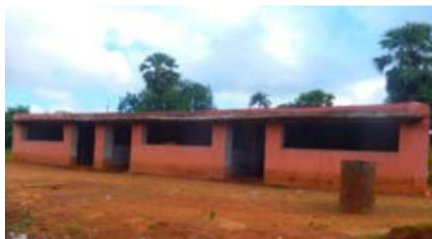
Newly constructed infrastructure
